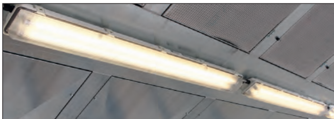
Plastic-Hanging lamp explosion protected for zone 2
